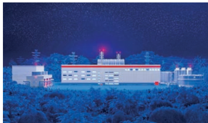
Land-based small modular reactor nuclear power plants
